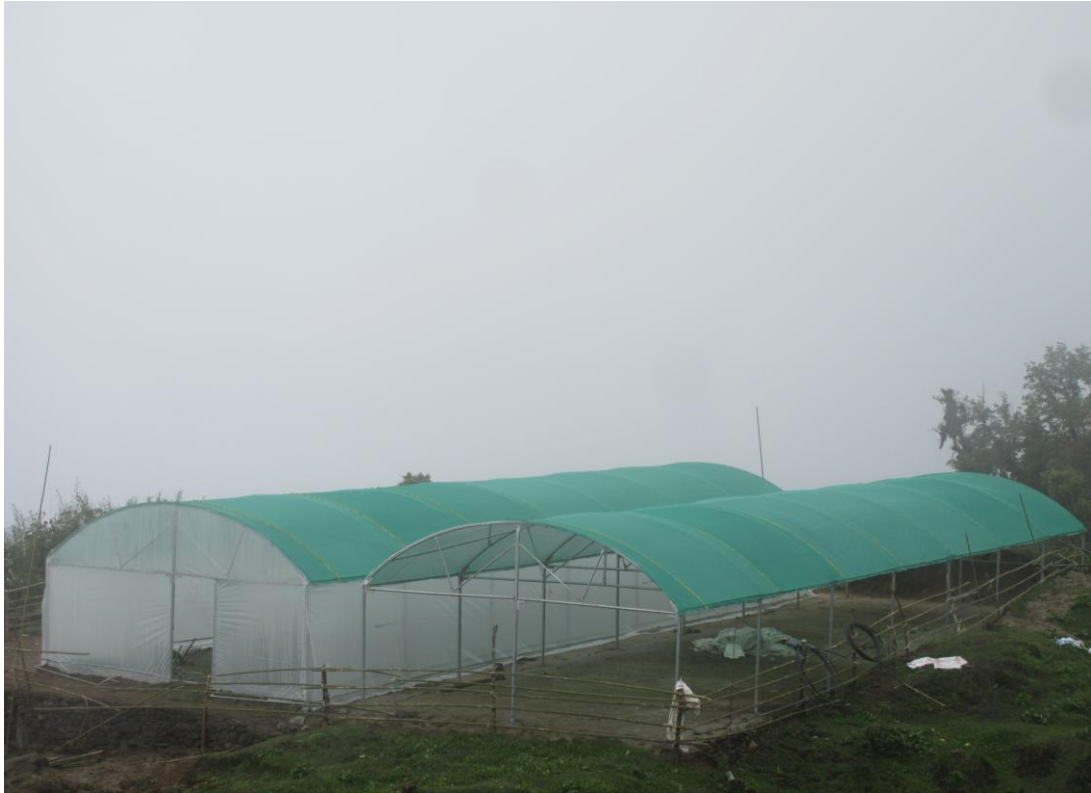
Photo 25: Photo of Greenhouse completed in Phungling-10, Phurubu, Bhalugaude
