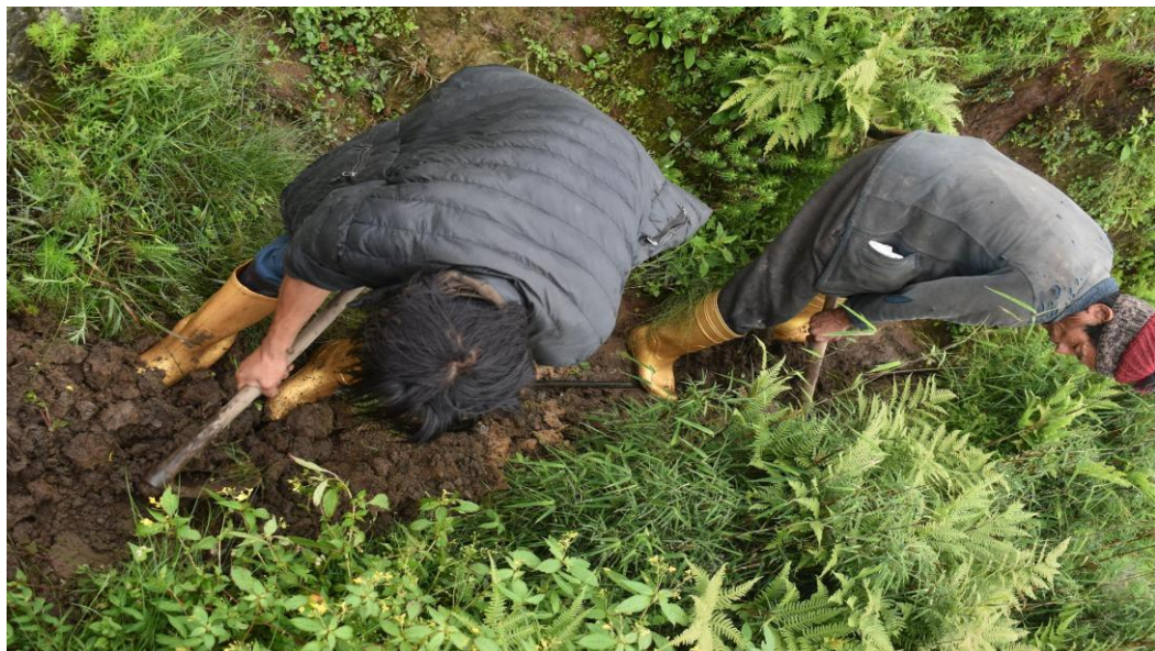
Photo 22: People carrying water pipe to Harkate
